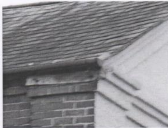
Tingles to slate roof
