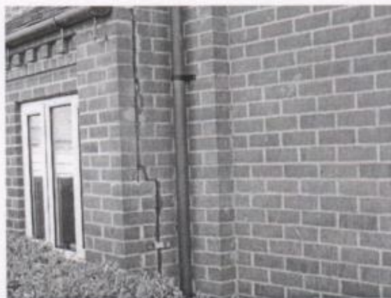
Vertical crack
