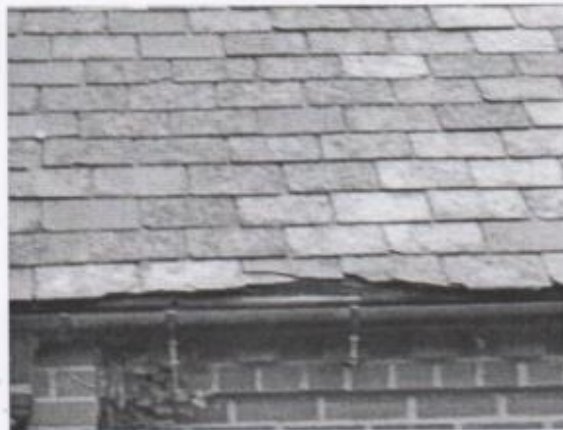
Damaged Slates
